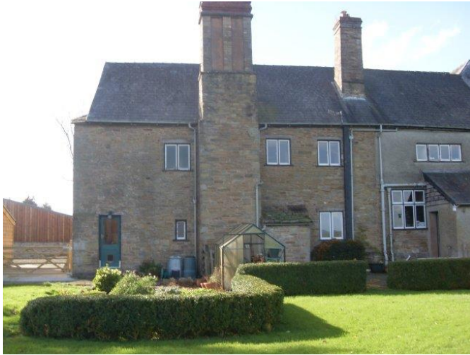
The East wing of Hergest Court
