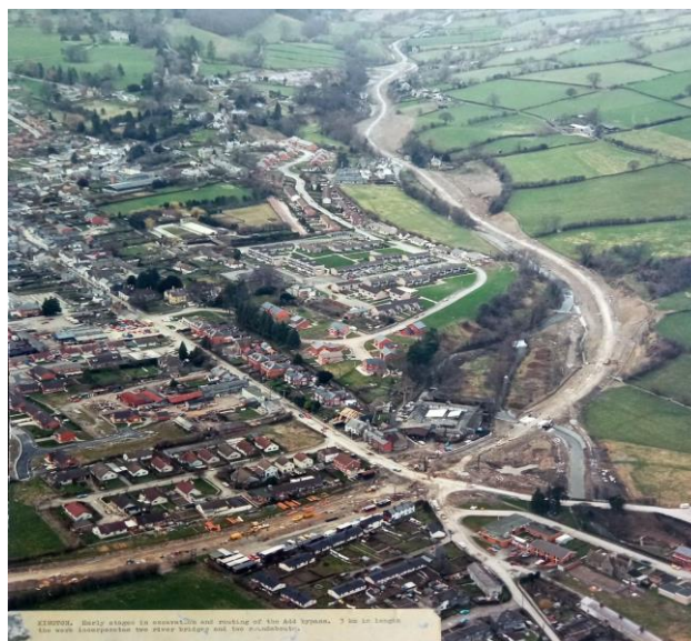
Aerial View of the Bypass under construction
