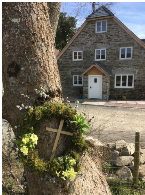
..... and after renovation
