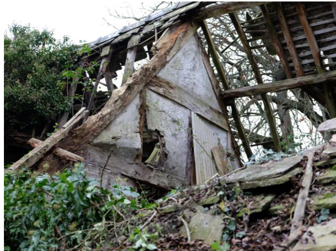
The mill before renovations
